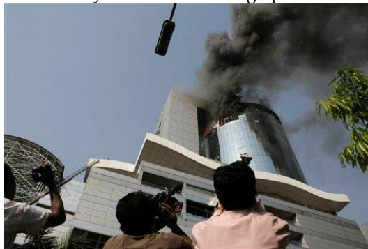
Figure 01: Fire in Bashundhara City Shopping Mall
