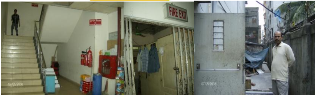
Fig 06: stair and fire exit
